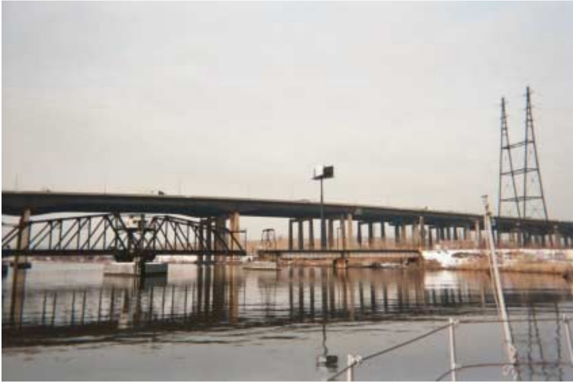
New Jersey Turnpike and Point-No-Point Conrail Bridges
